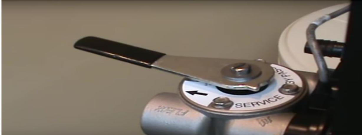
**Step 1:** Locate the level bypass valve.
